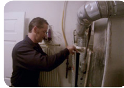
Furnace & Water Heater Inspection
