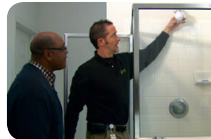
Energy Efficient Showerhead Installation
